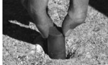
Magnets embedded in the ground guide vehicles along the roadway
